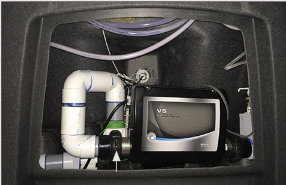
FIGURE 1.9 : HEATER UNION; LOOSEN UP TO BLEED AIR
