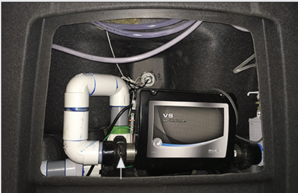
FIGURE 1.9 : HEATER UNION; LOOSEN UP TO BLEED AIR
